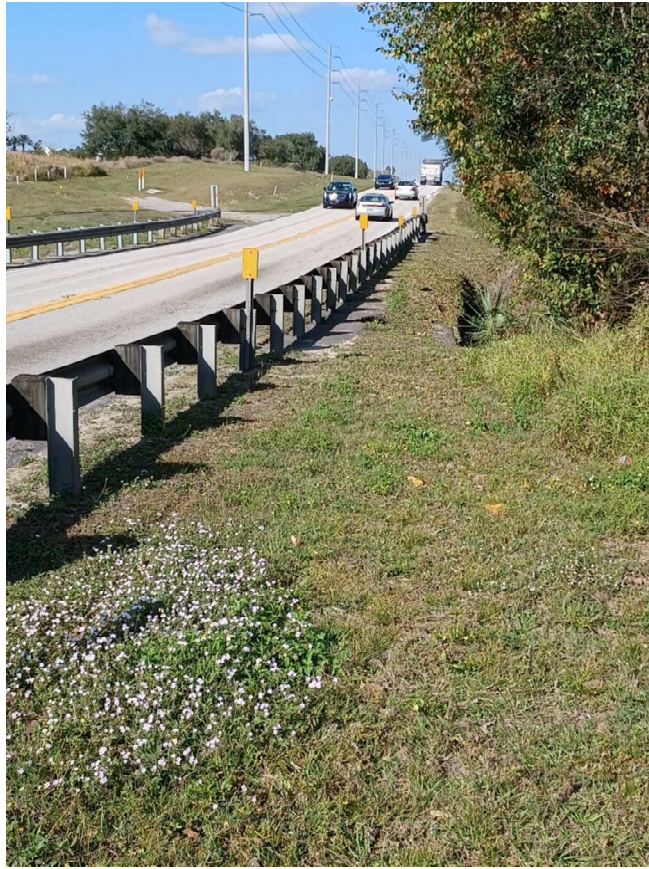
Photo 5: East side – Facing North
