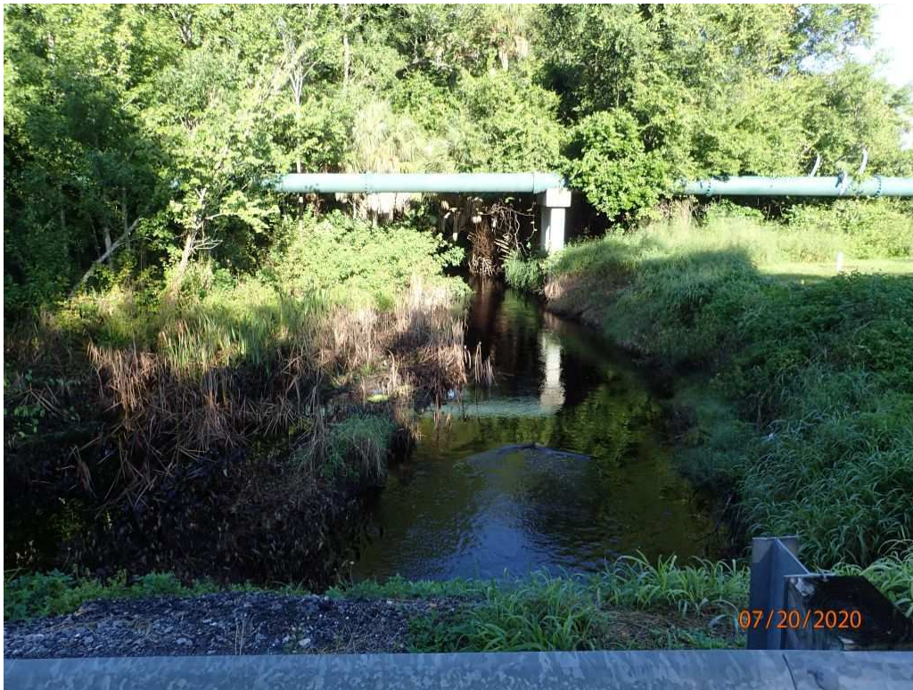
Channel Looking West
